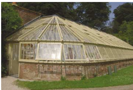
The completed vinery at Greenway (Kim Auston)
