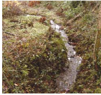
Cascades leading to partially silted up canal
