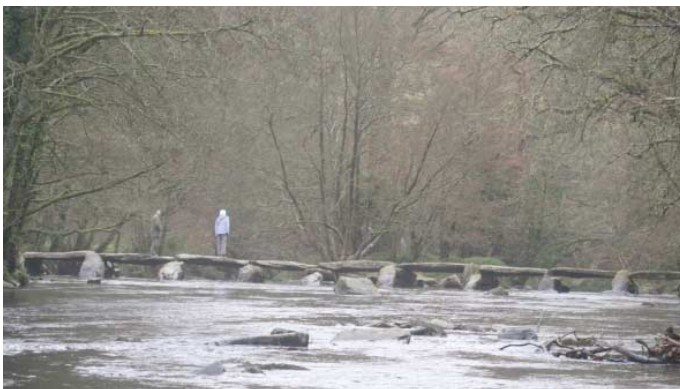
The clapper bridge at Tarr Steps (Rob Wilson-North)
