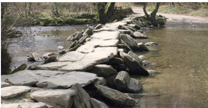
Close-up of the clapper bridge (Rob Wilson-North)
