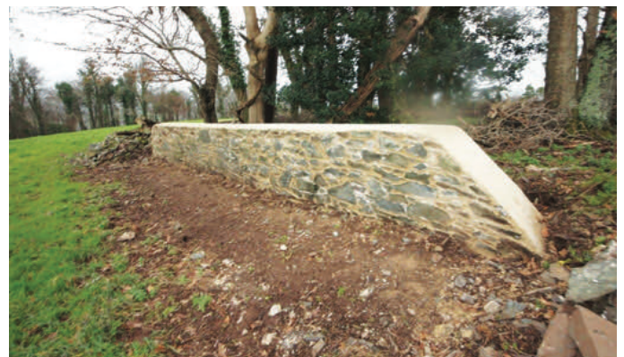
Figure 2. Left: the wall to this enclosure at Greenway was in a state of collapse. Right: following repair with Stewardship grant aid.
