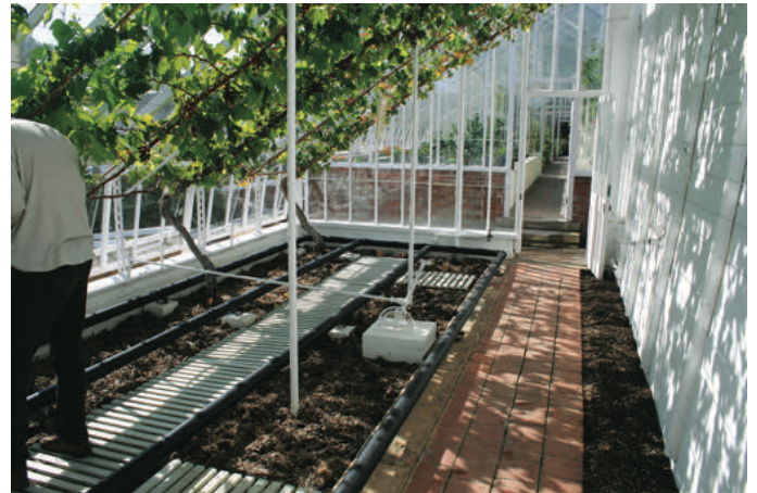
Above ground heating pipes and remote operating mechanism for front ventilators in a vinery
