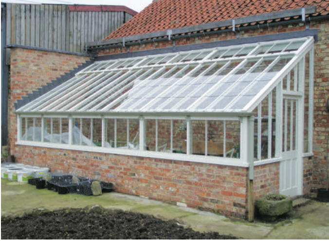
A lean-to conservatory with top-hung roof ventilator
