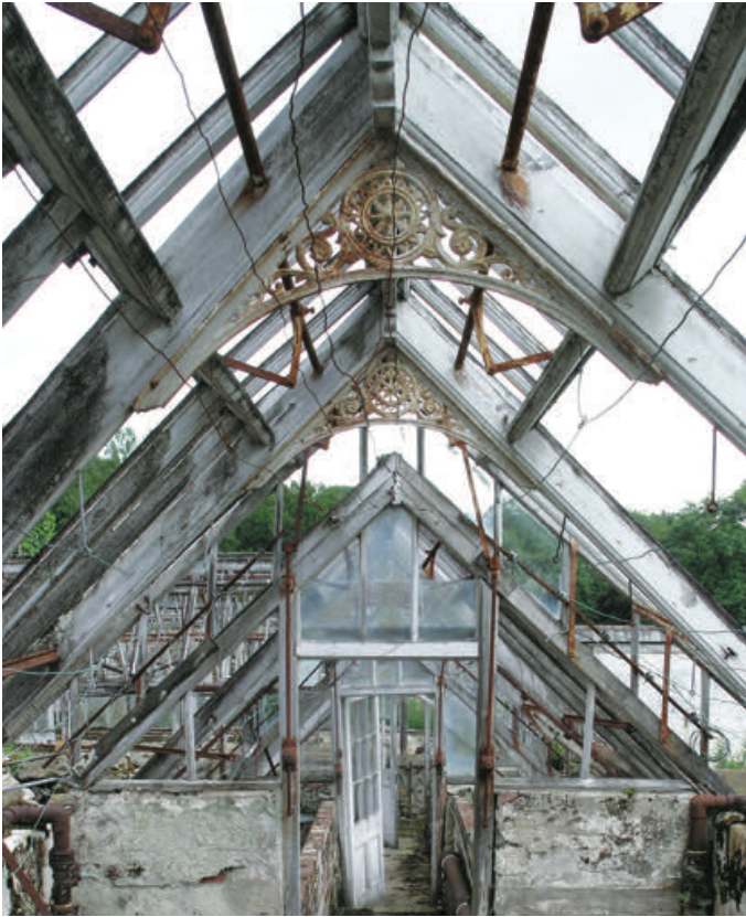
Abandoned glasshouses in Devon, showing fine cast iron spandrel brackets.
