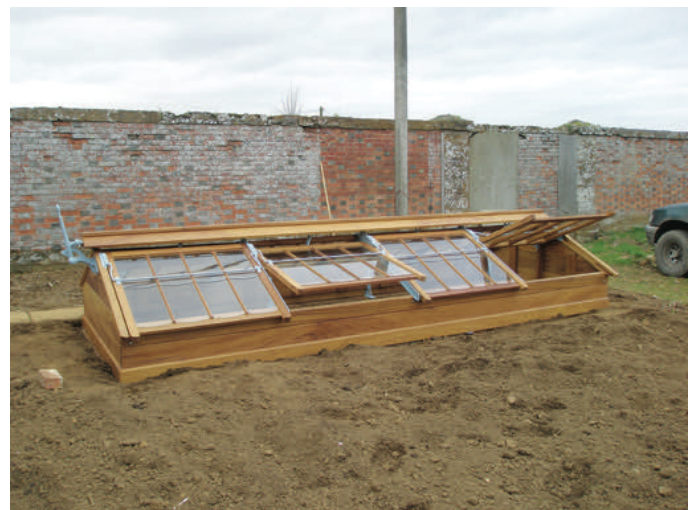
A new example of a Foster & Pearson clear-span cold frame with beaver tail glass. The lever at the end operates the ridge ventilator
