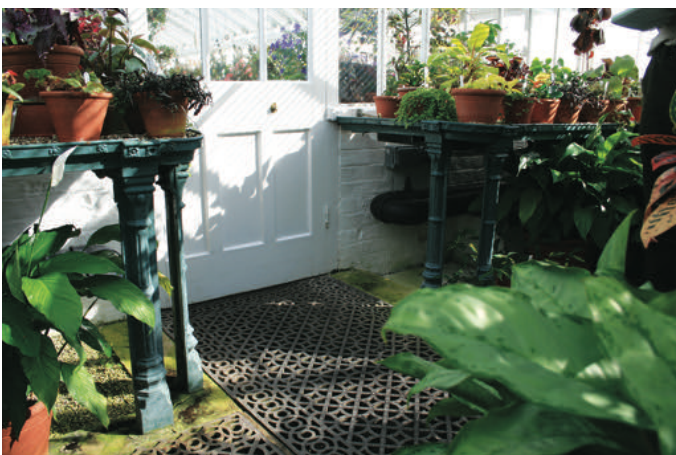
Cast iron staging with a grating below covering the cast iron hot water heating
