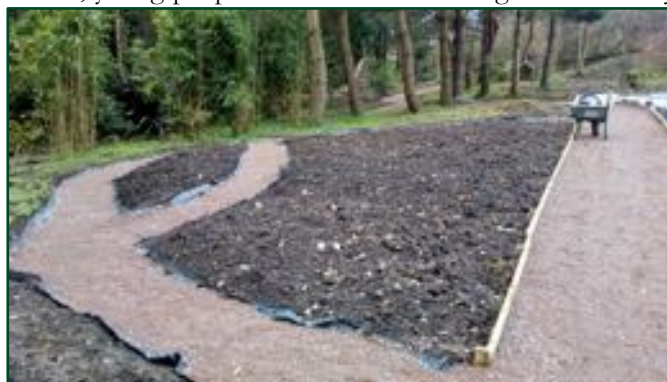
The WESC sensory garden under construction. © WESC
